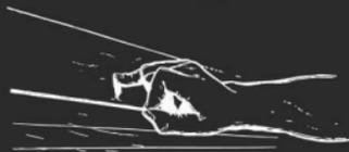
Snap an additional chalk line the width of a tile out from each wall. This will help keep the tile placement perfectly straight. Continue laying out tiles and spacers until placement is correct.
